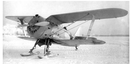
I-153 equipped with skids to start from snowy and frozen surfaces
